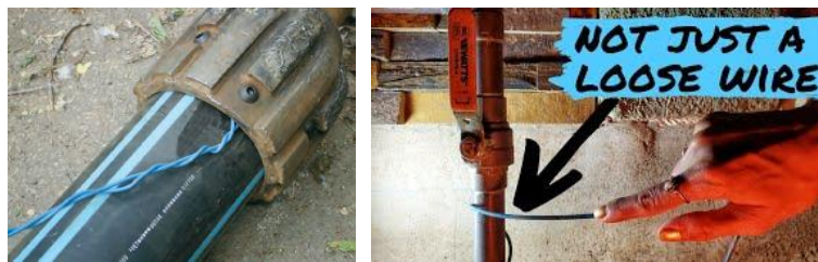
Figure 7 – “Blue” Tracer Wire
