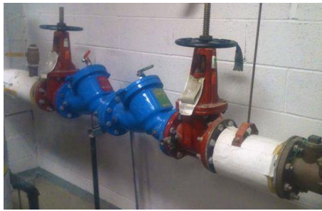
Figure 9 – Example of a Backflow Prevention Assembly
